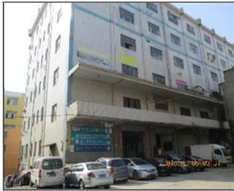
External photo(s) of the production unit(s) The factory building.JPG
