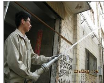
Photo of the inside of the main production hall Fire hydrant testing (2).jpg
